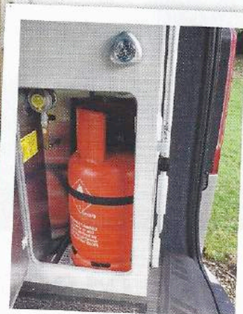
The LPG gas cylinder has its own locker at the back
